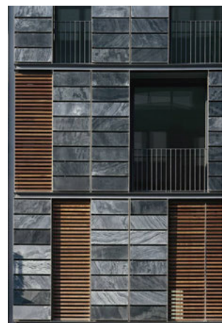
Housing building Balmes (OAB)
